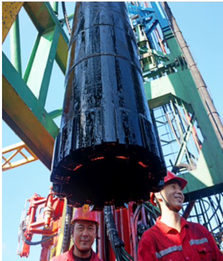
Drilling in the Songliao Basin in China reached a final depth of more than 7000 meter and sets several new records in ICDP drilling.
