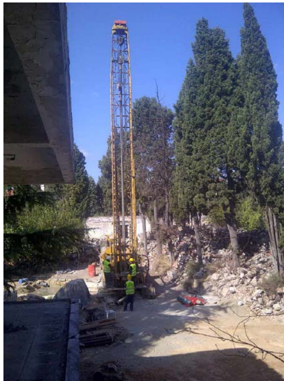
Spud-in for the first of eight boreholes of the Geophysical Observatory at the North Anatolian Fault
