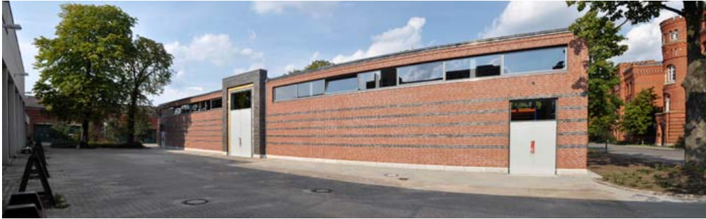
The new core repository at Berlin-Spandau was opened in September 2012
