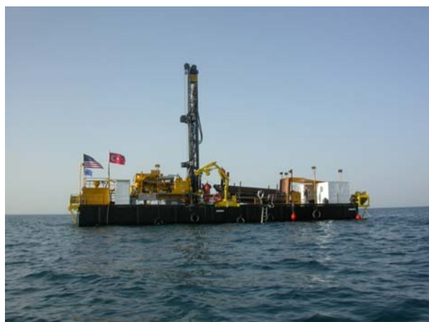
Figure 4: Lake Van Drilling in operation in July 2011
