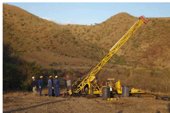
Drill rig at the Tjakastad site
