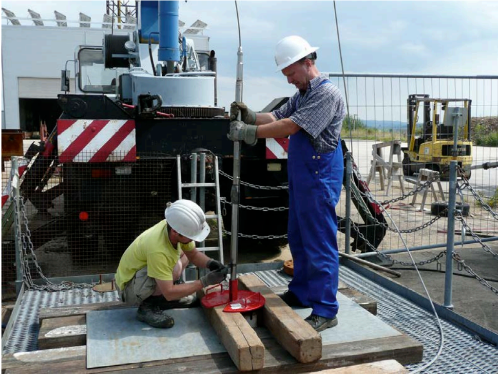
Installation of the SW geophone chain requires for a minimum of two specialists.
