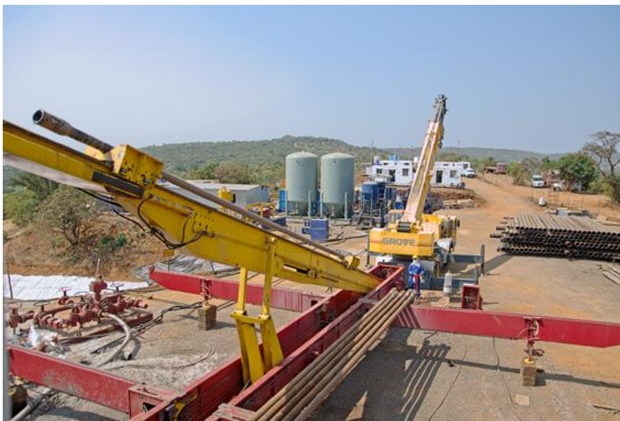
View from the rig floor during scientific drilling in Koyna, India, where a new drill pipe is lifted to the drill rig.
